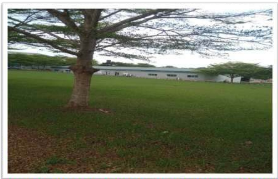
May & Baker Nigeria Plc's Factory premises in Ogun state.
